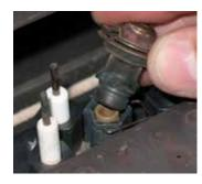
Unscrew the pilot orifice with the allen key; then replace with the LP pilot orifice
