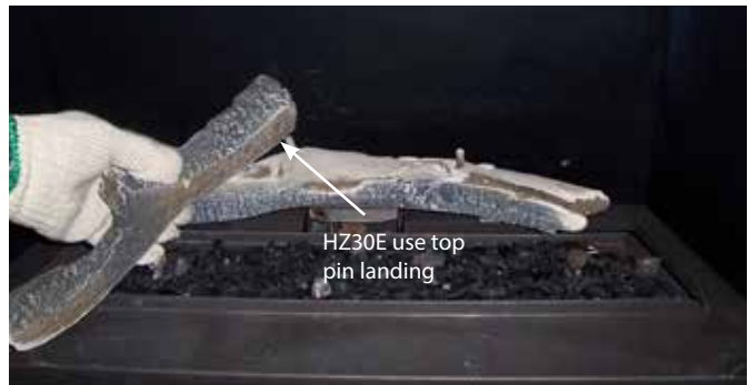
HZ30E shown - installing Log 2
