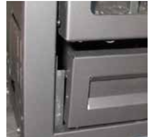
Installation of lower Flush Panel
