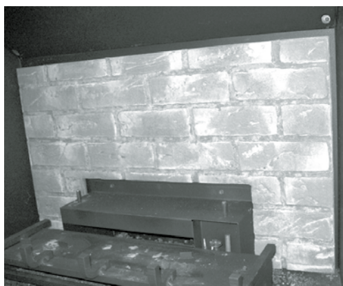
Back Panel Installed
